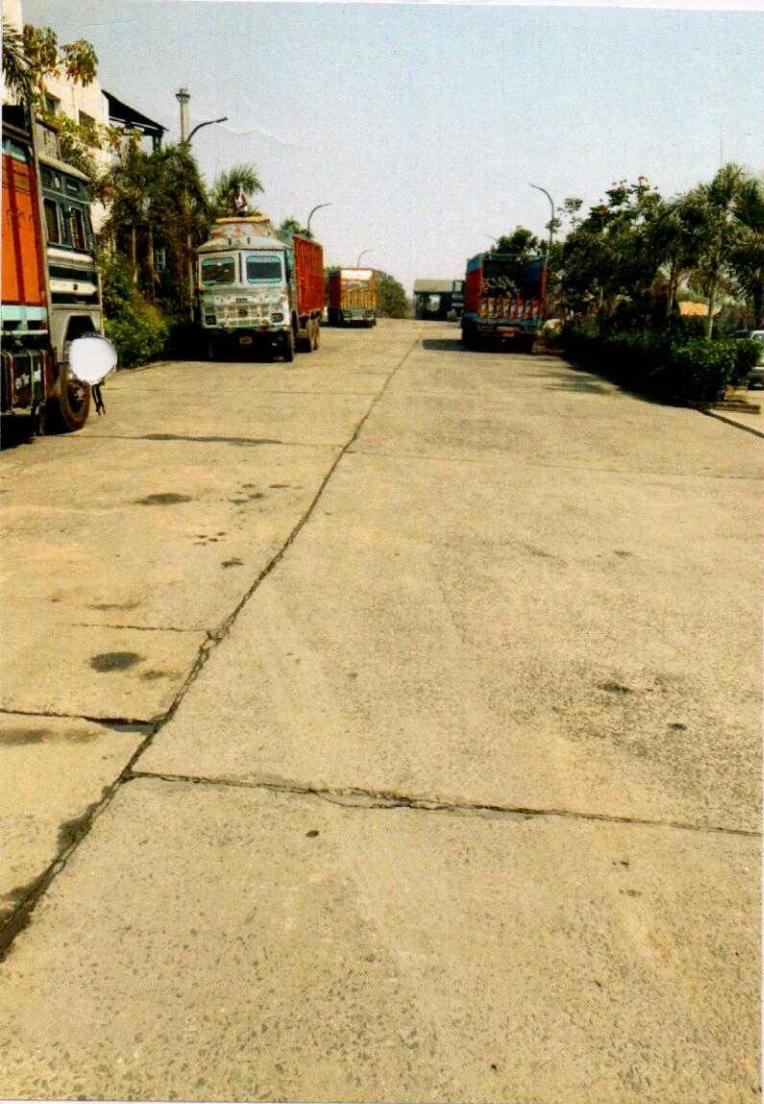
Photograph Showing Pucca Road all around inside Premises.
